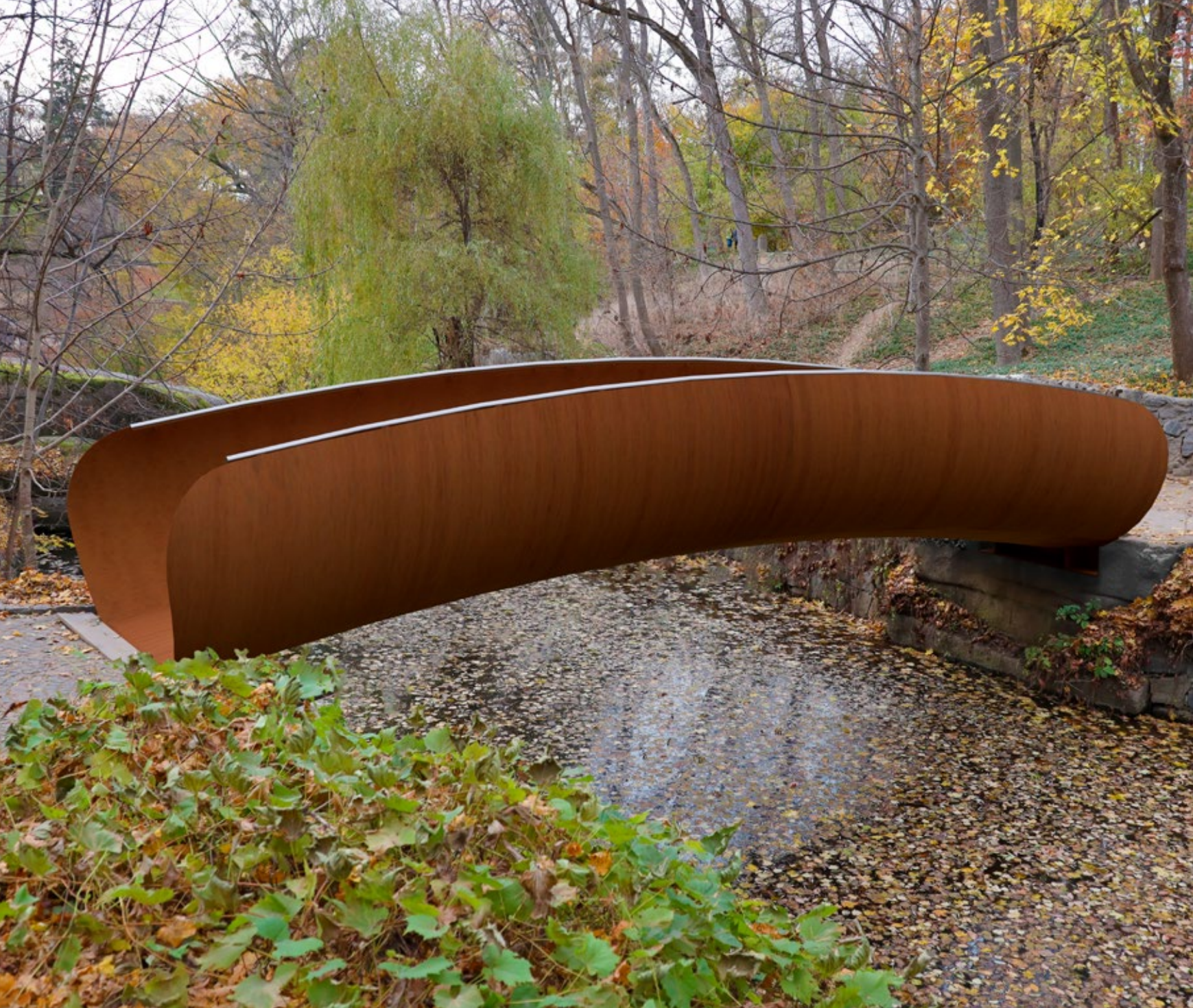
The Cocoon Bridge is a Corten steel bridge manufactured as a single, monolithic piece. This unique design is subtly arched and optimized for efficiency in its structural integrity.
