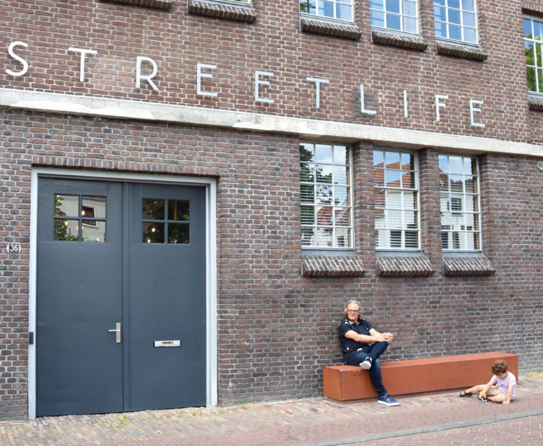
Streetlife runs its operations from a monumental industrial warehouse in the heart of the city of Leiden (NL). The Wolpakhuis dates from 1929 and has been completely renovated under the supervision of our own construction team. Historical details have been preserved and the building's authentic industrial character has been combined with modern technology and comfort.
